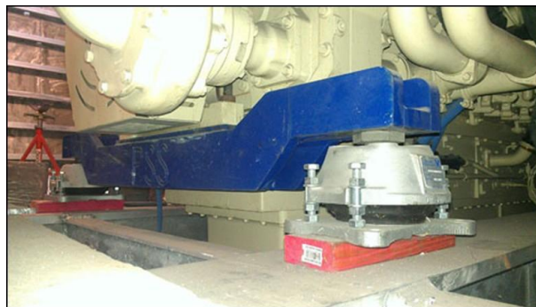
FIGURE 5-7 RESILIENT MOUNTINGS
